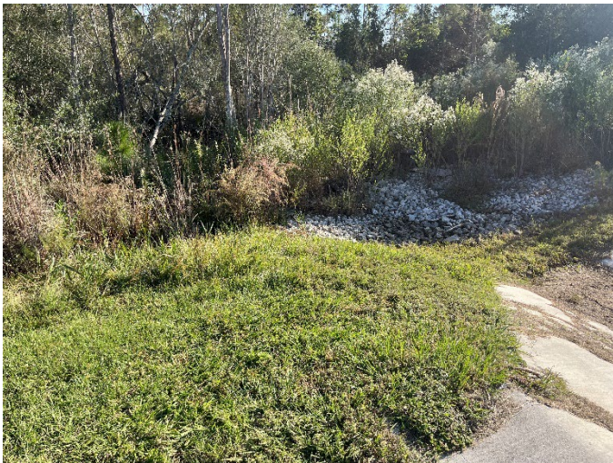
P-15C Riprap at Outfall Structure.
