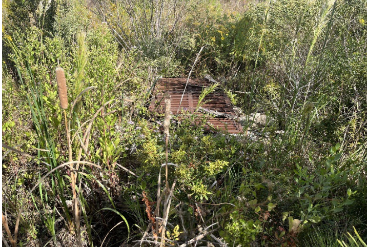
P-14D Entrance Culvert
