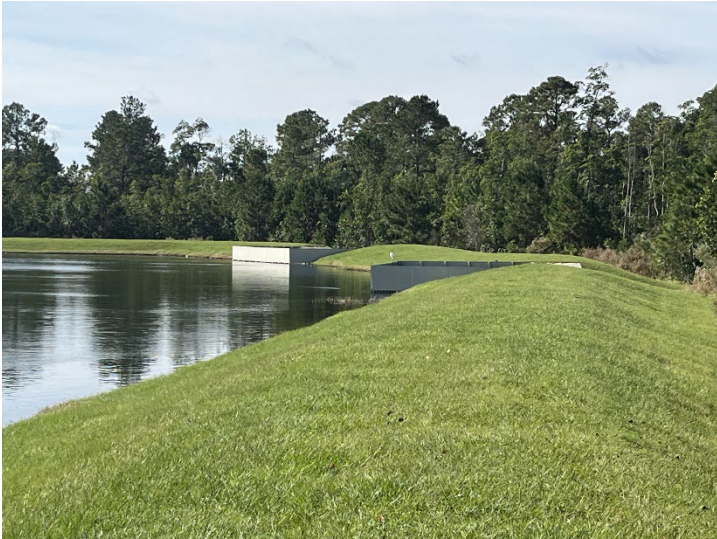
P-1 Outfall Structure Spillway #1 (Foreground) and Spillway #2 (Beyond)
