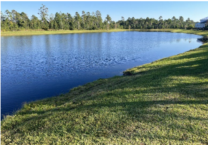
P-10 View Facing South
